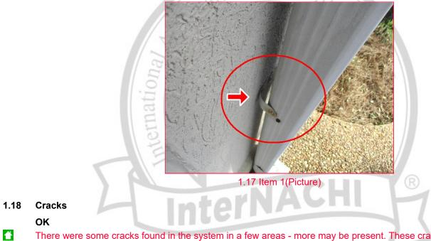
There were some cracks found in the system in a few areas - more may be present. These cracks need to be sealed to protect the integrity of the system.
