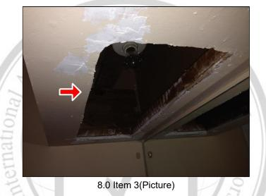
(4) Repair plumbing leak and replace damaged tile.
