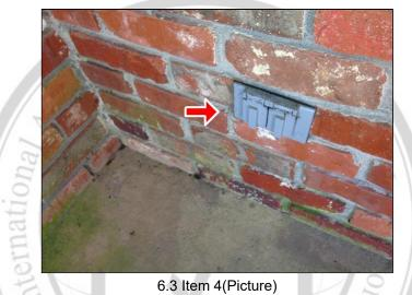
(4) Wires under kitchen sink need to be in a make up box.
